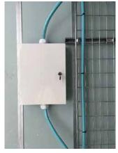
FIBRE OPTIC BREAKOUT BOX INSTALLED WITHIN TENANT'S RISER
